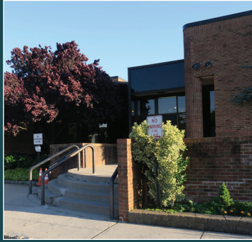
Bridgewater branch 1 Vogt Drive Bridgewater, NJ 08807 (908) 458-8415
